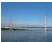
Audubon Bridge (USA)
